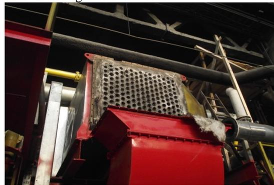
**Fig.5 View of the air pre-heater, from the flue gas entrance side towards the damaged tubesheet**
