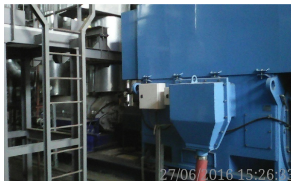
Fig. 1. The electric motor and pump No. 3
