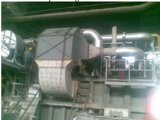
Fig.4 View of the air pre-heater while mounting it on the aluminum scrap melting furnace
